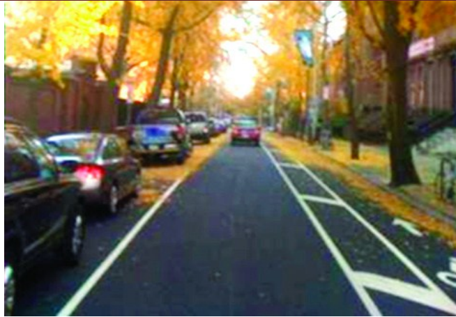
Figure 2.7 the lane width for motor vehicle travel was reduced to provide exclusive space for cyclists (Source: Relationship of Lane Width to Safety for Urban and Suburban Roadways, 2007).
