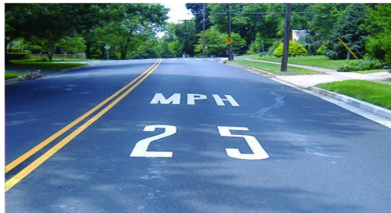
Figure 2.5 Special pavements marking to encourage speed reduction for impending curve (Source: Handbook of Road Safety Measures, 2004).
