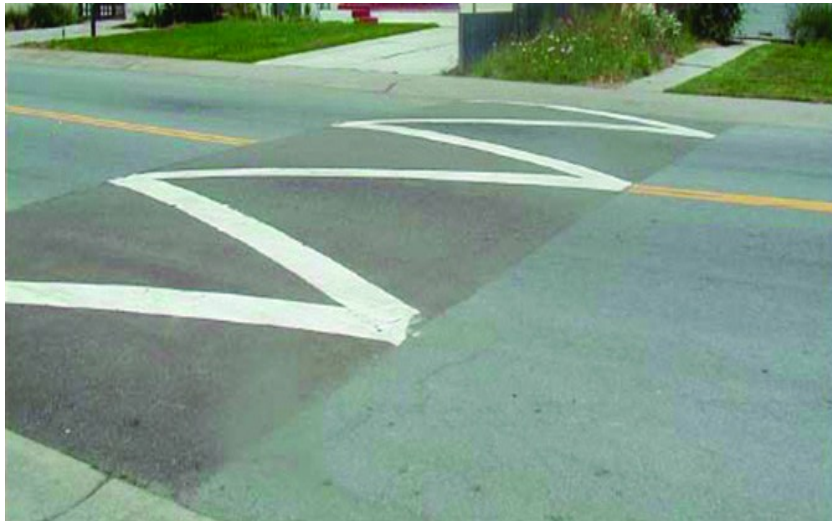
Figure 2.9 a speed hump delineated to notify motor vehicles of its presence (Source: Speed Management Guidebook, 2012).
