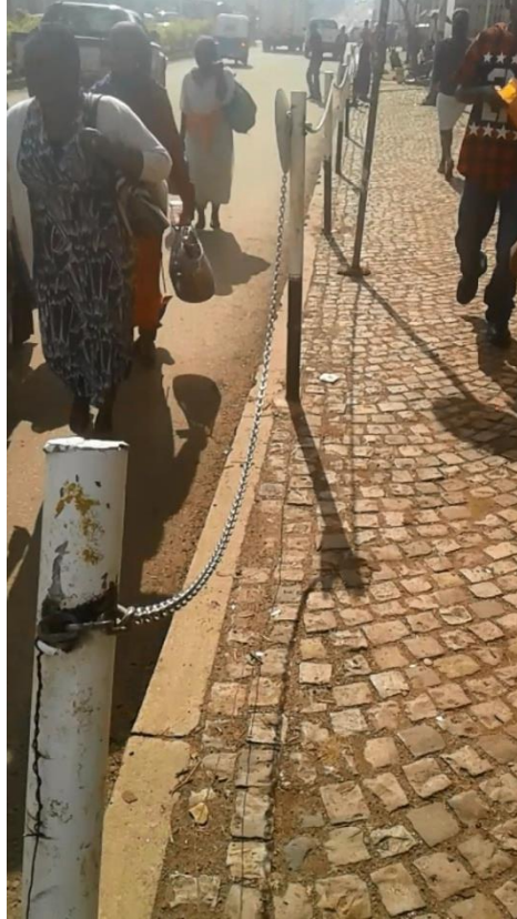
Figure 3-18: Barrier at the Road Side of Pedestrian Walkway
