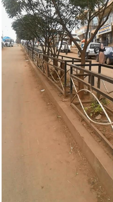
Figure 3-20: Trapezoidal Ditch at Areboch Tera – Jebena
