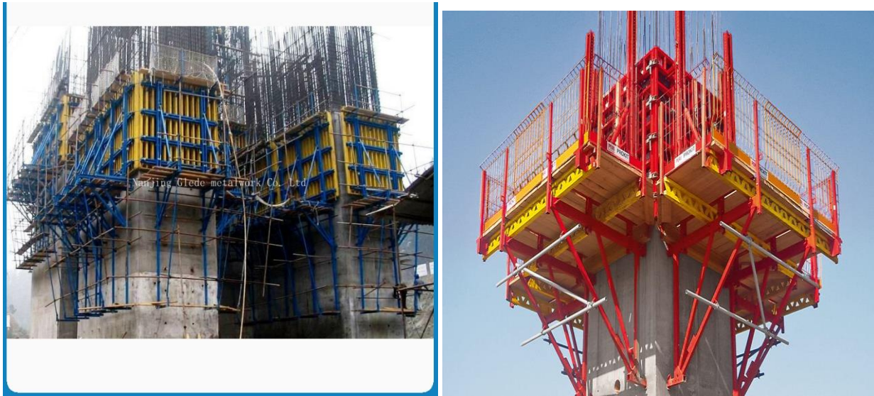
Figure 2.13 Jump or climbing formwork [14]
