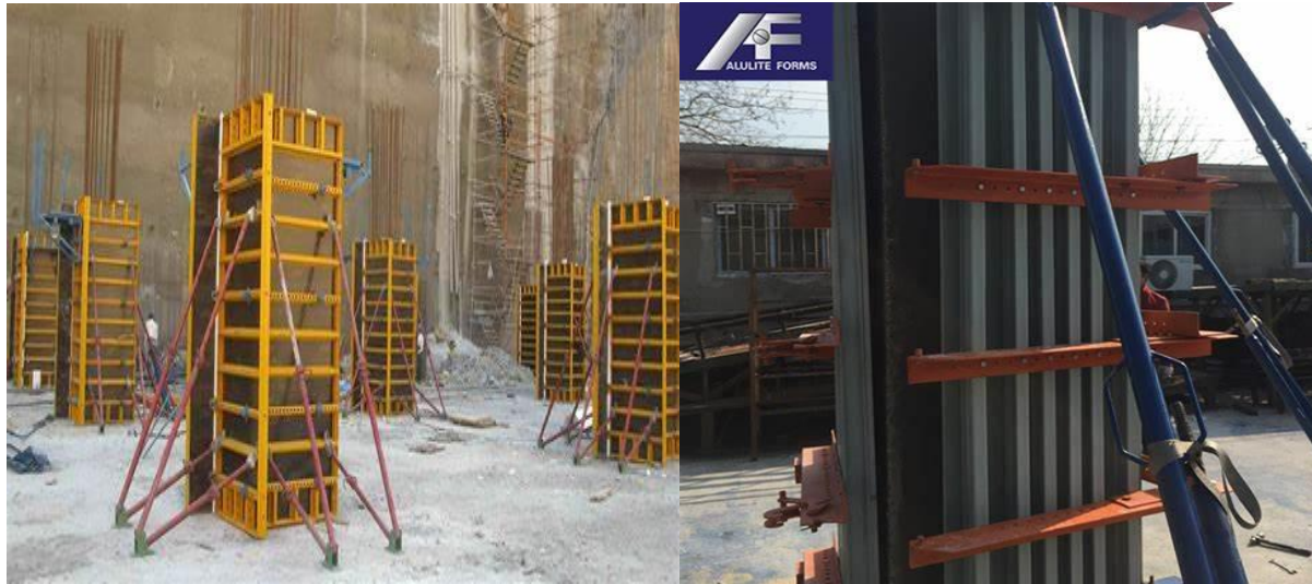
Figure 2.10 Column formwork system [14]
