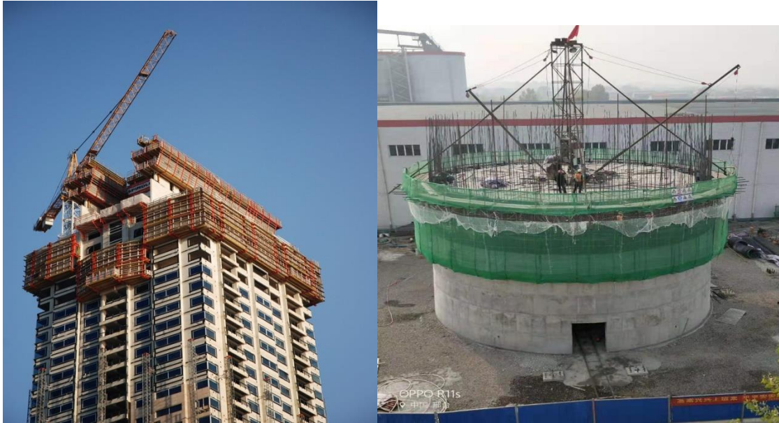
Figure 2.14 Slip Formwork System [14]
