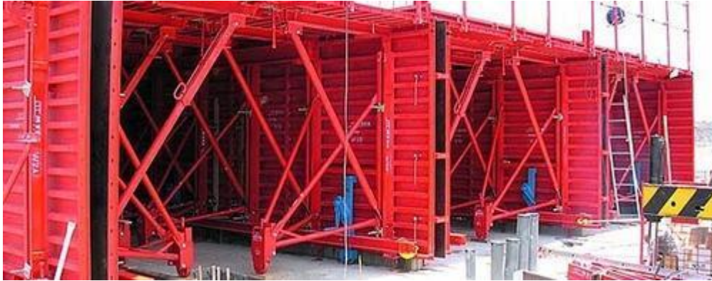
Figure 2.15 Tunnel formwork system [14]
