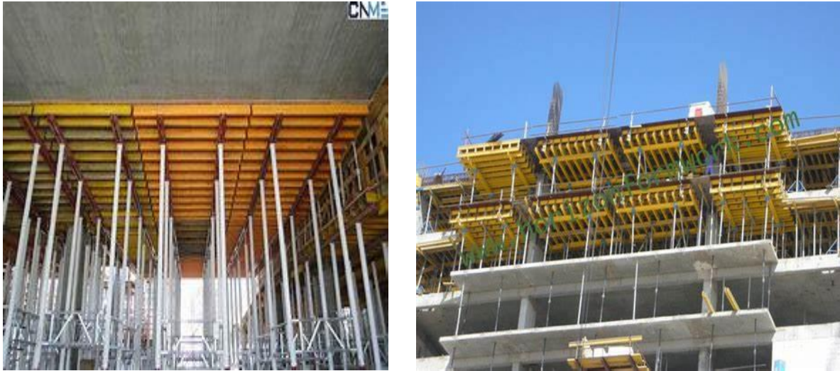
Figure 2.9 Table or flying formwork system [14]
