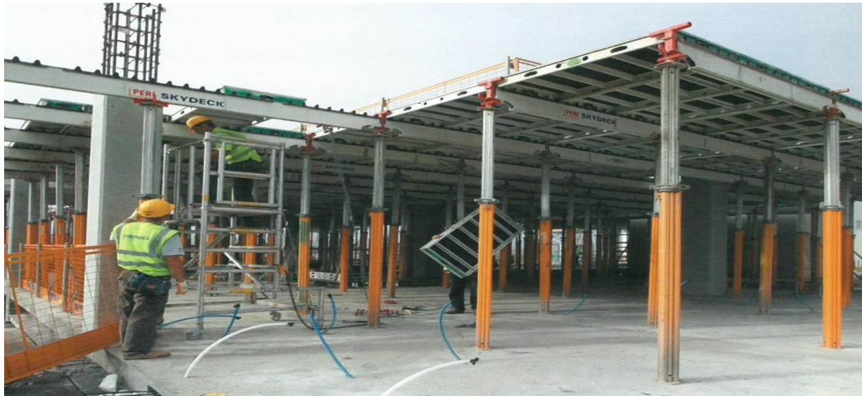
Figure 2.11 Horizontal panel system [14]
