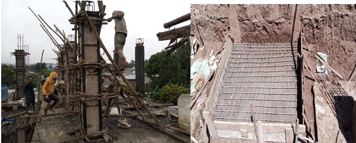
Figure 2.7 Conventional formwork system
