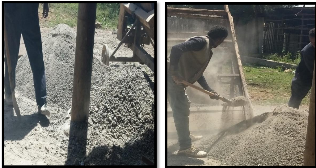
Figure 6: Extraction of fine aggregate from demolished HCB wastes
