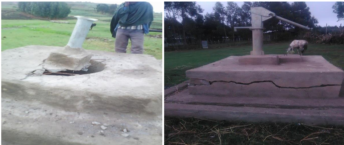
Figure 4: The construction quality of removal of spare parts and cracking of non-functional water supply points in the study area (source: field observation, July 2015)
