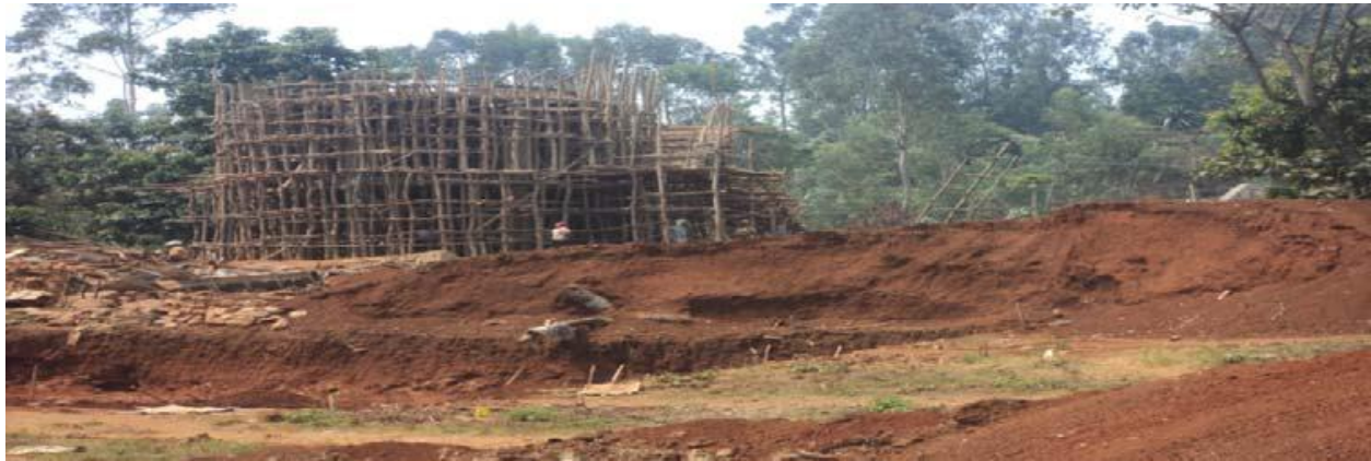
Figure 4-9:Metu town water supply under construction
