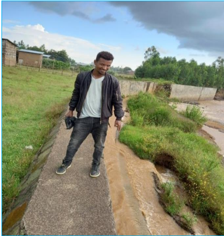
Figure 4.5 overtopping of canal
