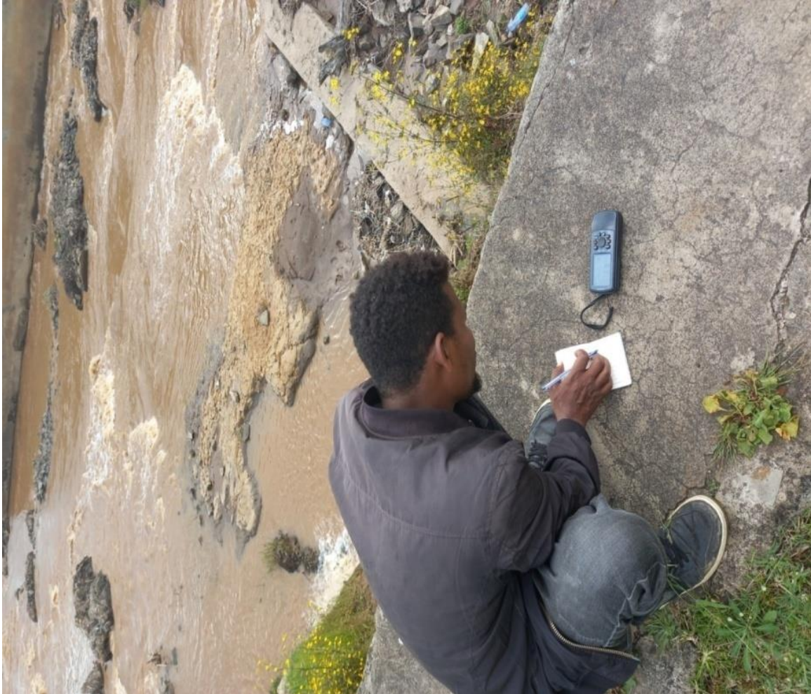
Figure 4.2 damage of downstream apron
