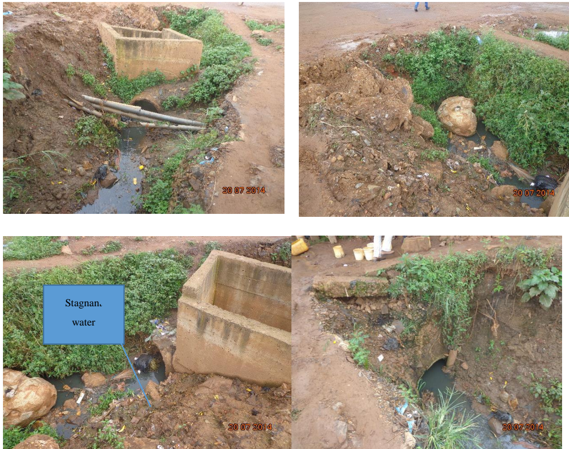
Figure 3.2Photos of Existing Drainage around Bus Station
