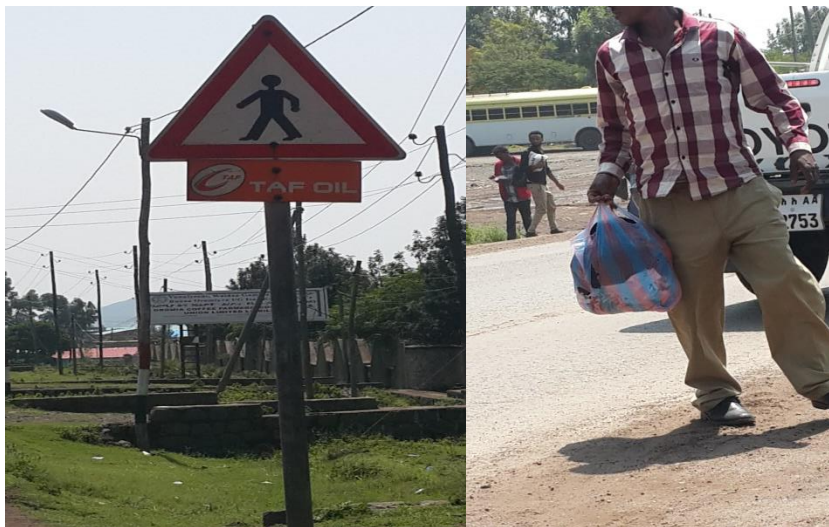
Photos 4.2: Pedestrian crossing at Gelan with faded zebra
