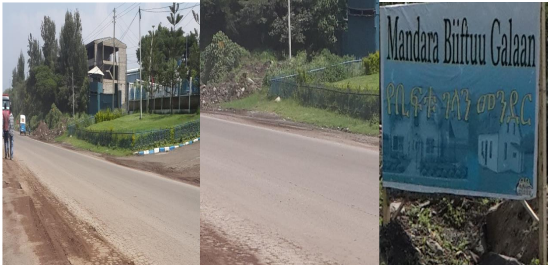
Photos 4.1: Problem observed up to Galan exit on installed safety devices
