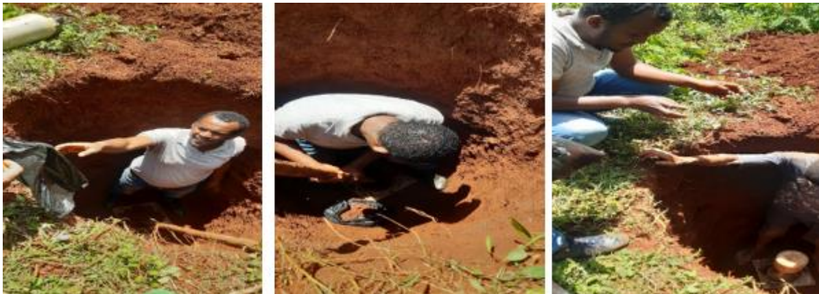
Sampling and conducting of sand cone tests
