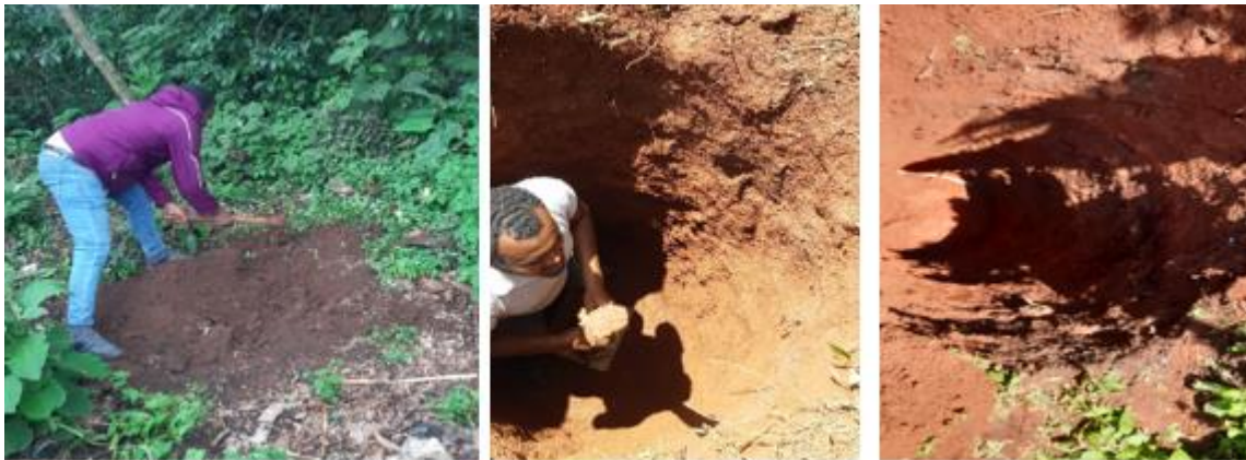
Excavations of test pits
