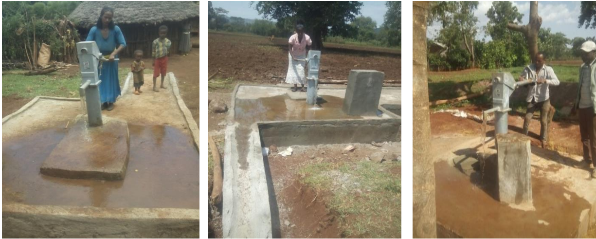
Figure 2. Selected Picture illustrating Hand pump and Hand dug well in the study area.
