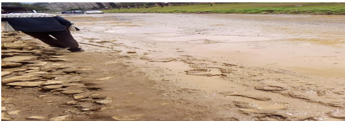
Figure 4. 2. Half and/or Full Part of the Road Occupied with Water and Mud [Photo taken by Researcher on July, 2022]
