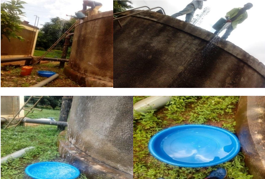
Figure 10: Spray aerator from groundwater
