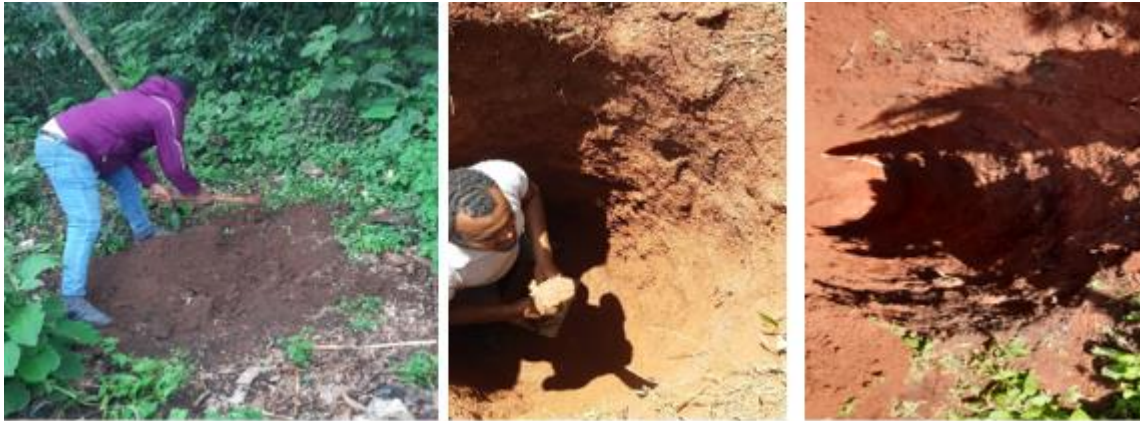
Excavations of test pits
