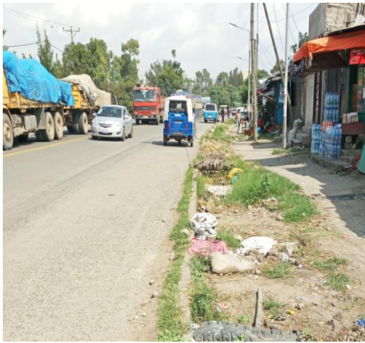
Poor condition of curb stone
