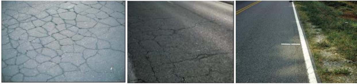
Fatigue Cracking
