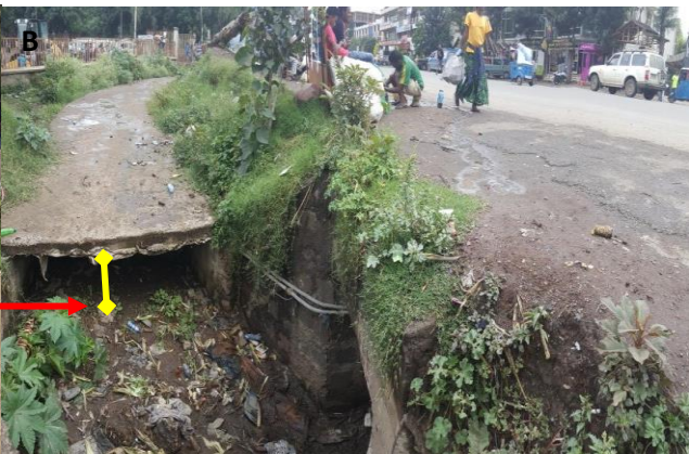
Drainage line in front of bus station seriously blocked with silt-up of mud and waste
