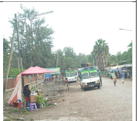
Flood prone area with no side drainage
