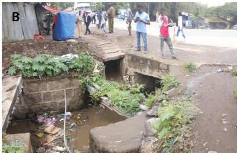
Outlet point of highway culvert
