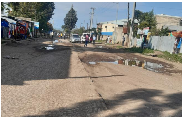
Road Profile condition during no rain
