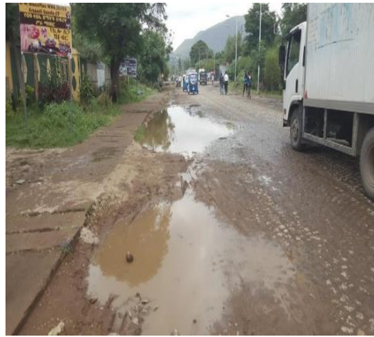
Slab cover not receiving surface runoff
