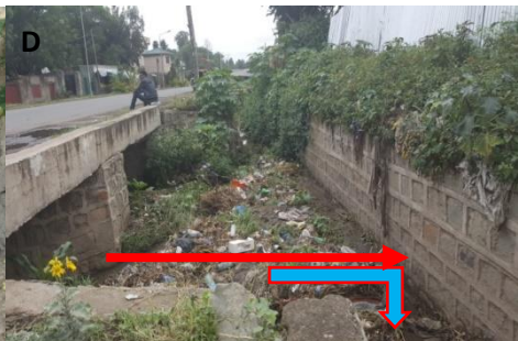
Wall in front of outlet
