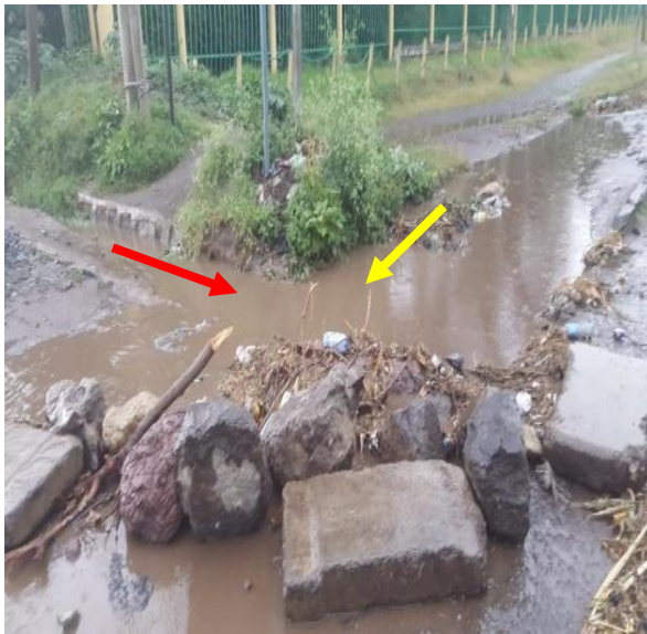
Closed slab culvert condition
