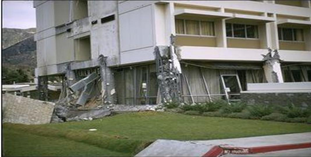
Figure 1.1a Failure of Olive View Medical State Center (Moehle and Mahin, Nisee Berkeley)
