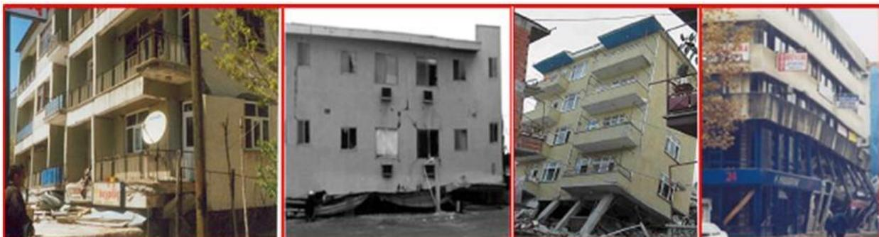
Figure 1.1b Failure of buildings due to soft storey in Turkey during Sumatra earthquake 2004 (Kirac et al. 2011)
