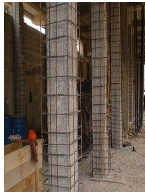
Figure 2.5: Construction techniques for column jacketing ( Safeguard your structure by Column Jacketing , no date)
