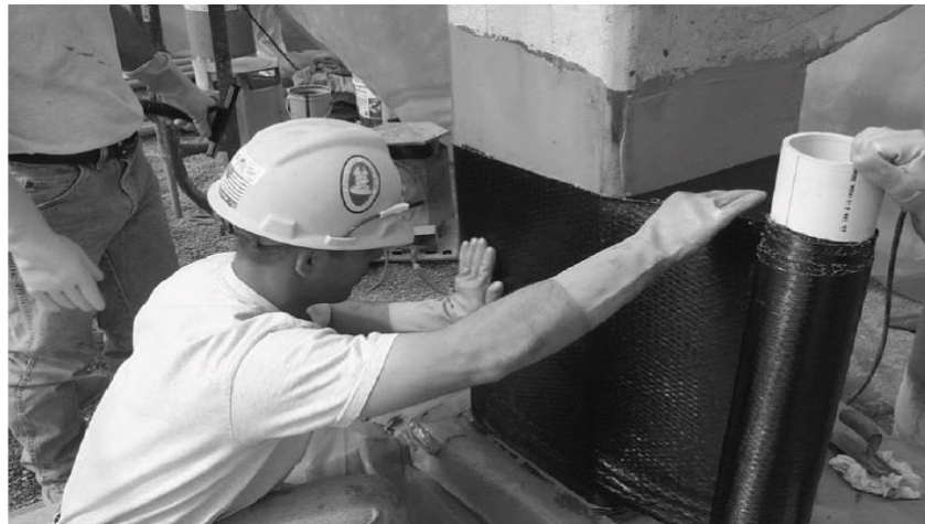
Figure 2.3: Installation of FRP wraps(AL-ALAILY, 2011)
