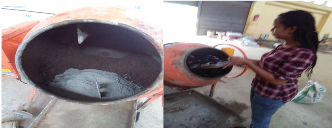
Photo:- mixing concrete
