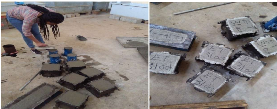
Photo:compacting and finishing mold concrete
