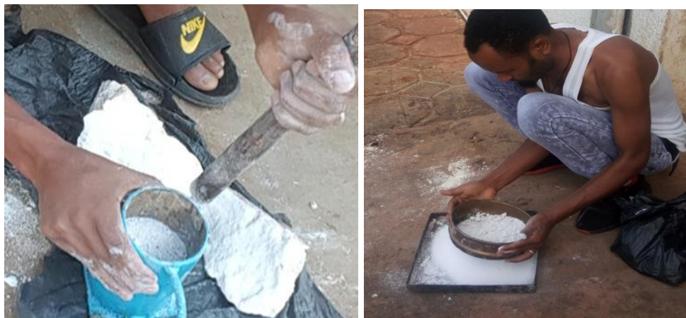
Figure 3.2: Preparation of Lime (photo taken by Anteneh)
