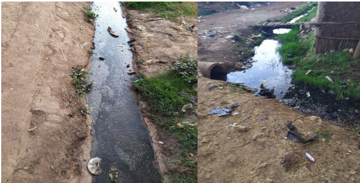
Figure 4. 6: Stagnant flood that occurs due to insufficient slope provision
