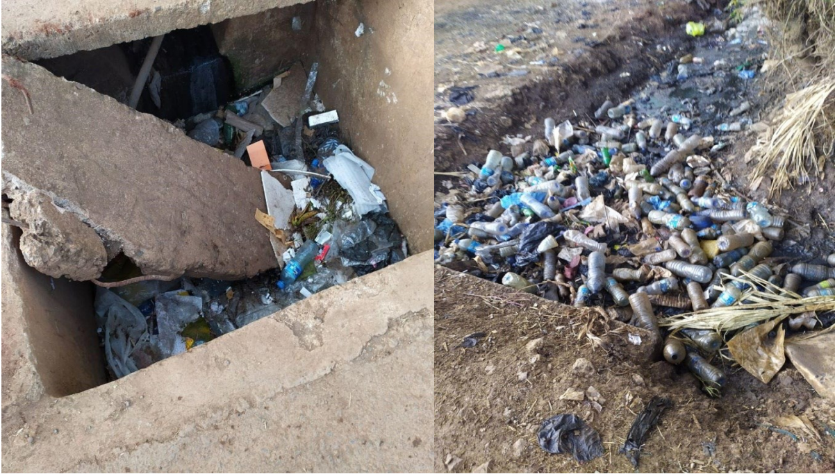
Figure 4. 7: A typical ditch covered by domestic solid wastes.
