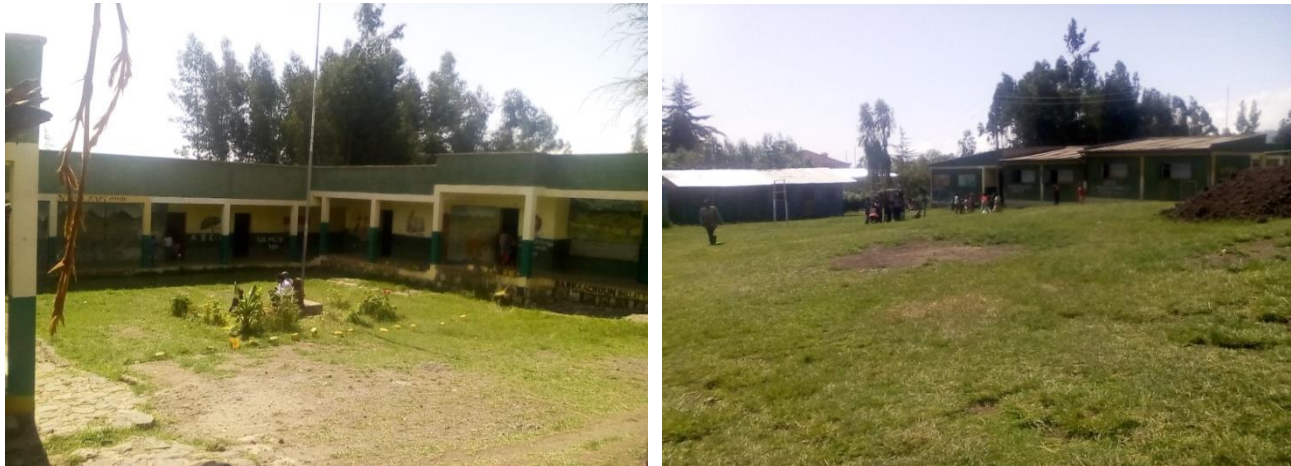
Fig.13. Partial view of the former the Gobba Child Caring Institution and the today's Mädehané'alām Kindergarten and Primary School
