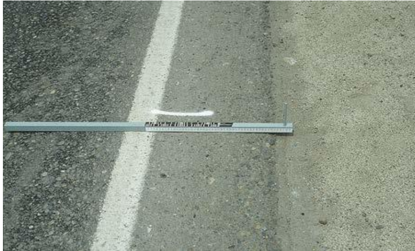
Figure 2-5 Lane-to-Shoulder Drop-Off(22)(28)
