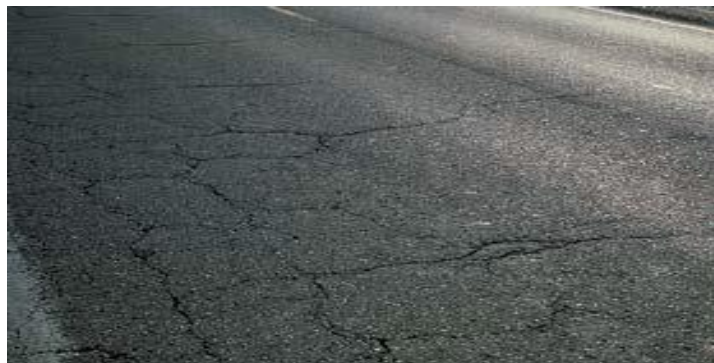
Figure 2-3 Block Cracking(22)(25)
