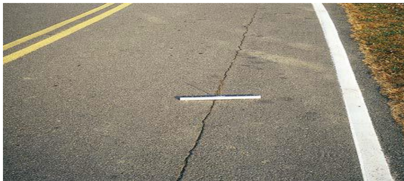
Figure 2-6 Longitudinal Cracking(22)(28)
