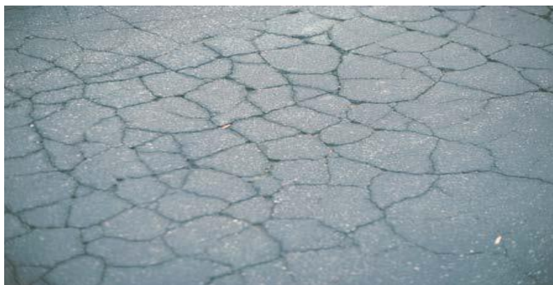
Figure 2-2 Fatigue Cracking (22)(25)
