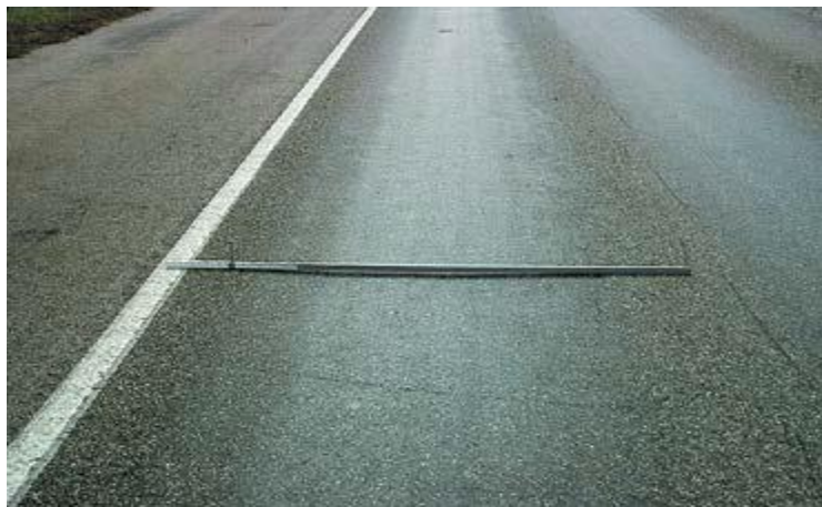
Figure 2-8.Rutting (22)
