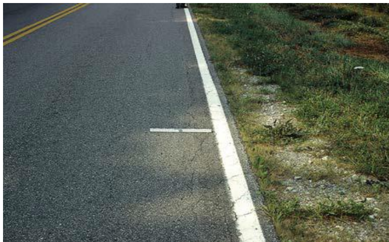
Figure 2-4 Edge Cracking(22)
