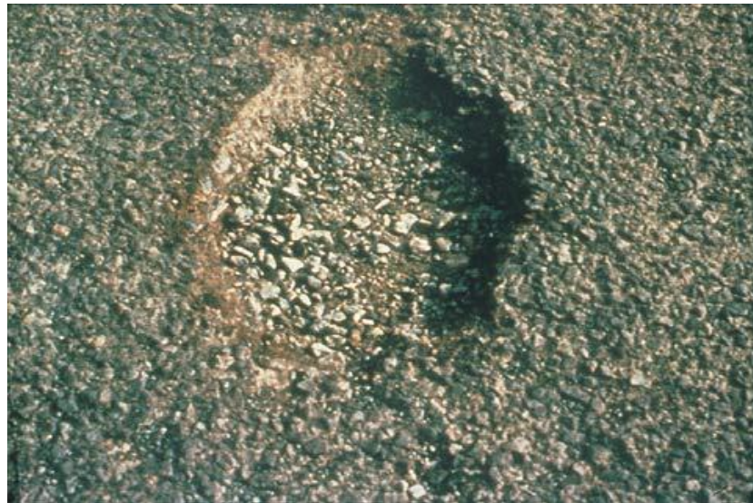
Figure .2-7 potholes (22)
