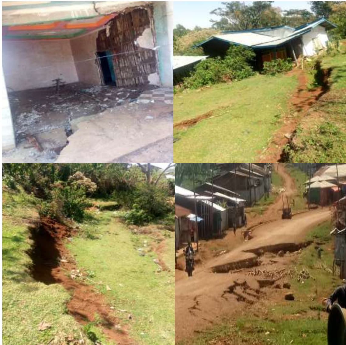
Figure 4.16 Some Photos on Consequences of Chira Town Landslide
