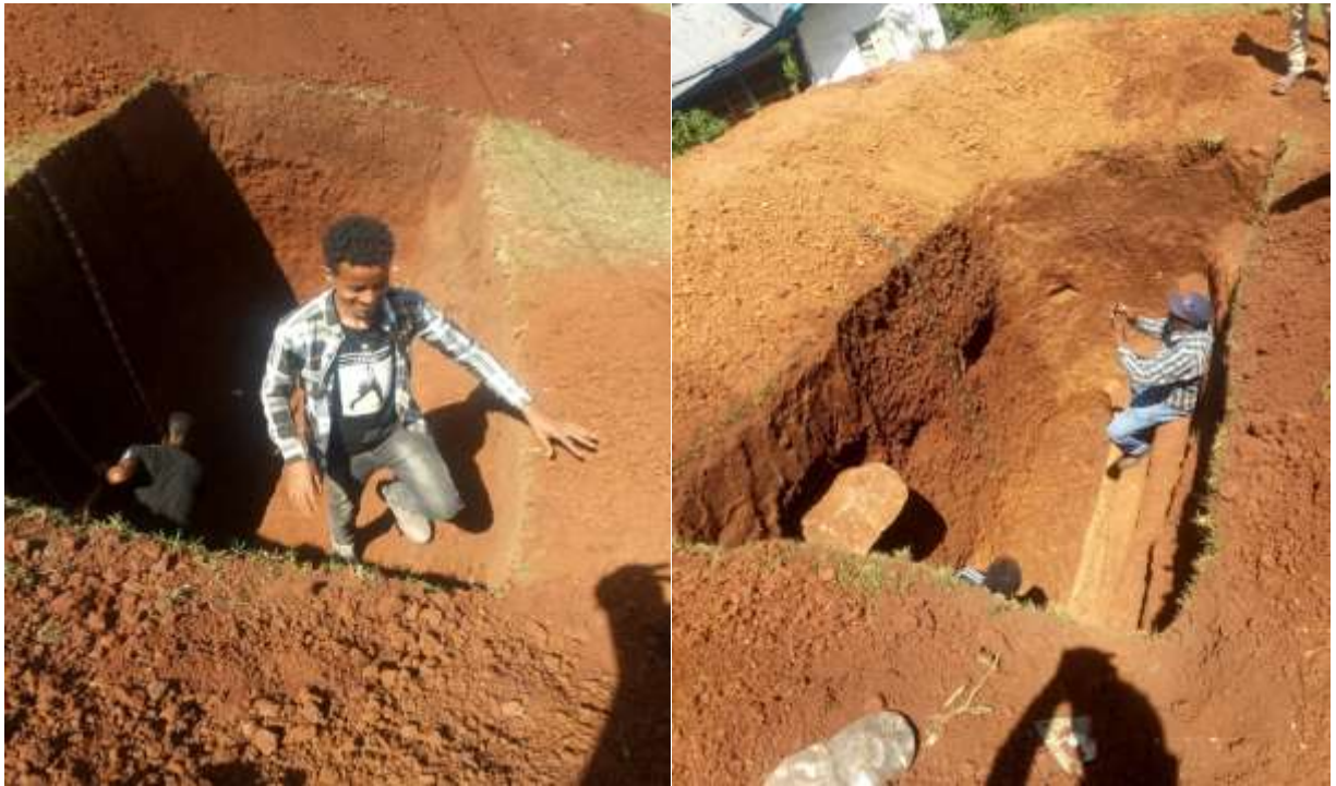
Figure D2. Photos taken during boring test pit.
