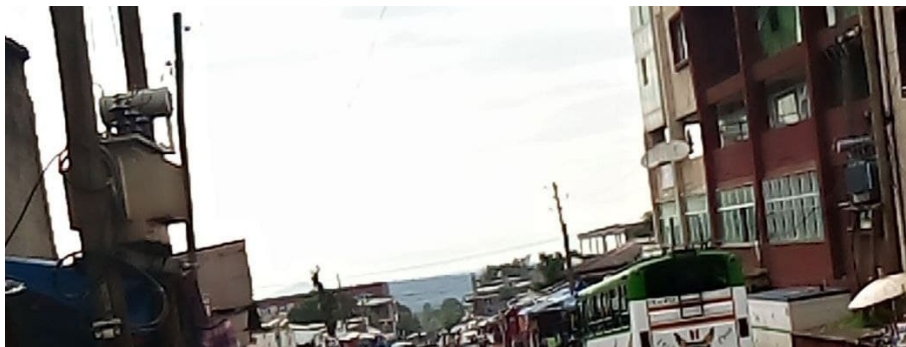
Figure 4.9: Photos for Dilla town distribution trafo.
