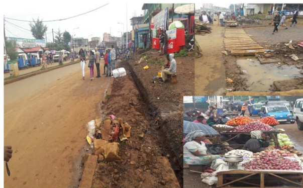
Fig. 3.1: Sidewalk quality problem, absence of buffer and presence of illegal occupancy on walkway in Nekemte city
