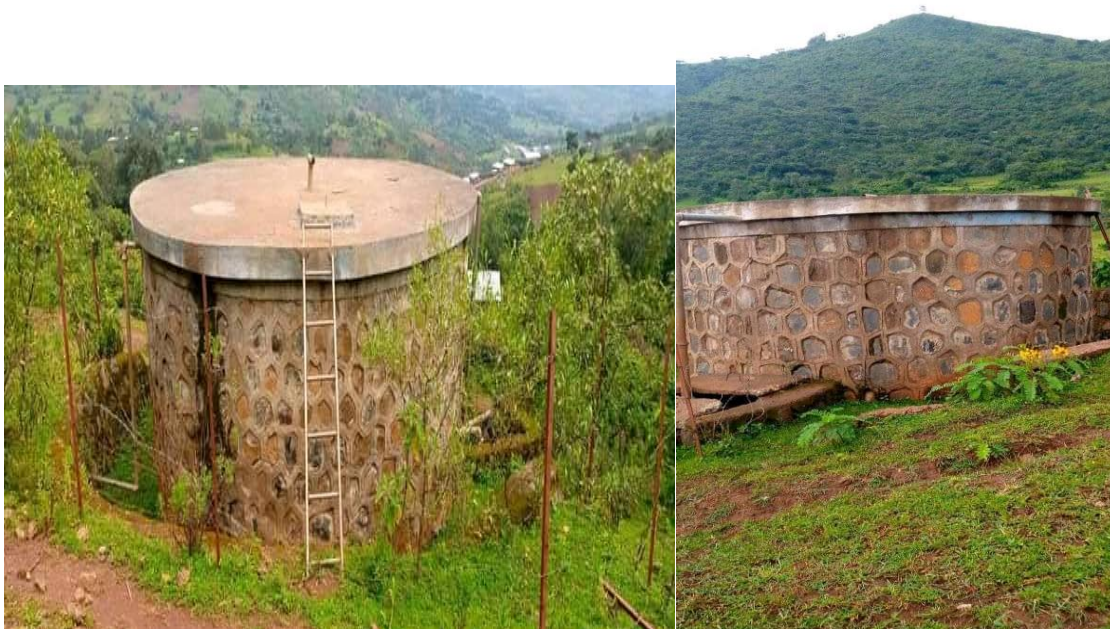
Figure 4.2 Sample figure of service reservoirs
