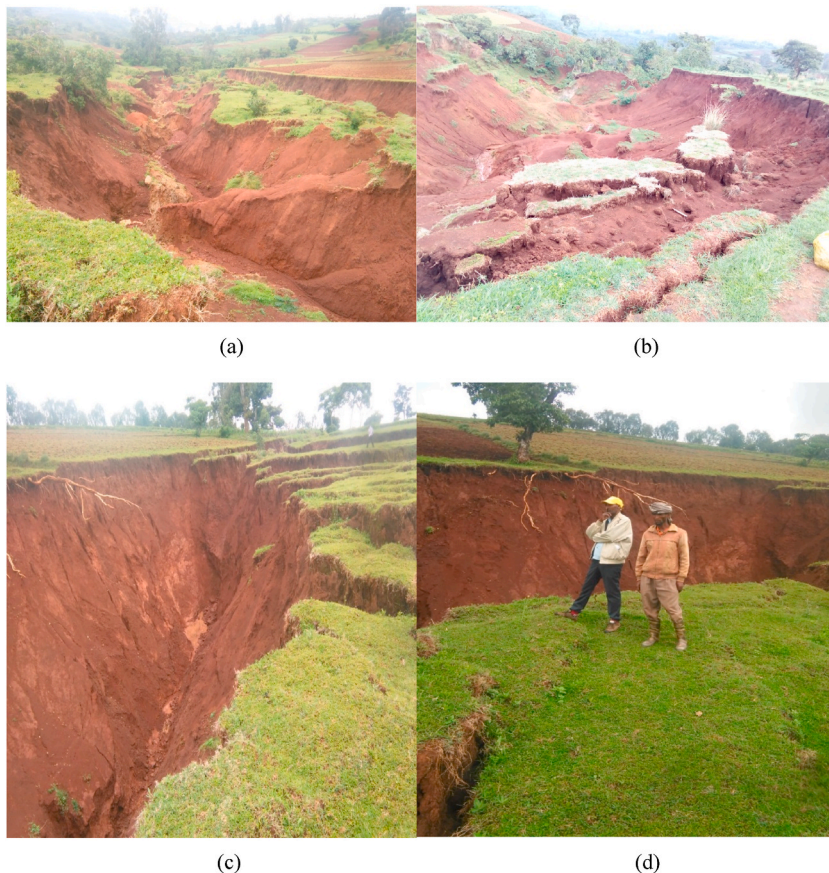
Fig. 2. Photo captures of the site indicating down ward and outward movement of soil mass.
