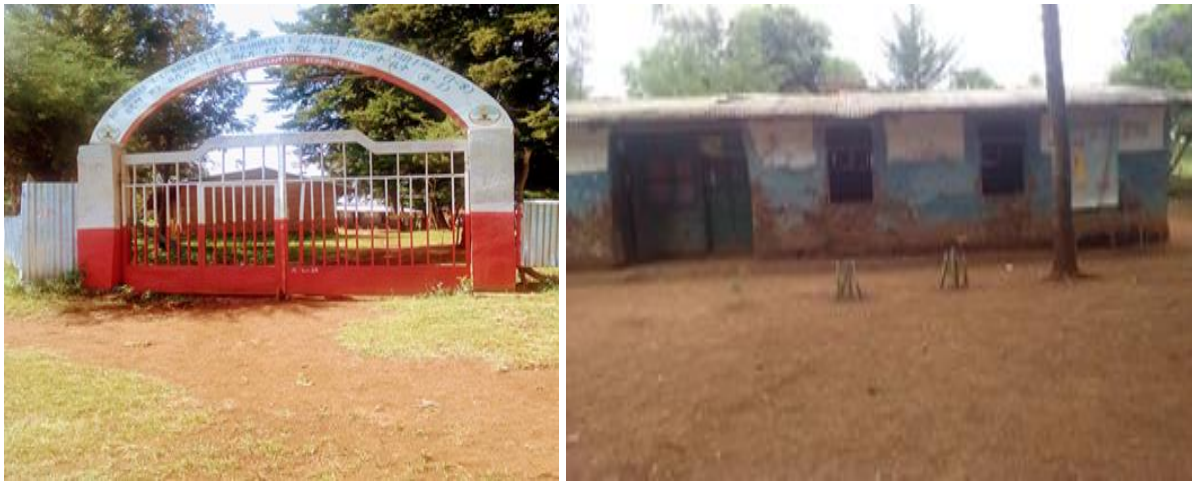
Figure 6: The First Building Standing Still of Gena Dire Elementary School
