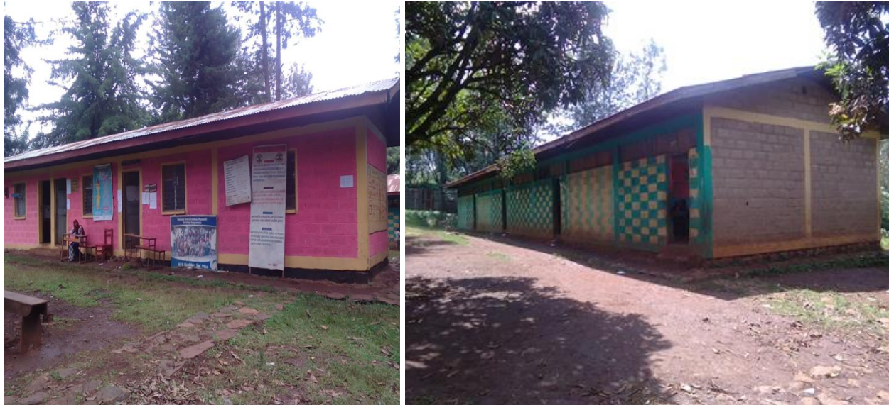
Figure 4: The First Babu Elementary School Rebuilding the former classroom
