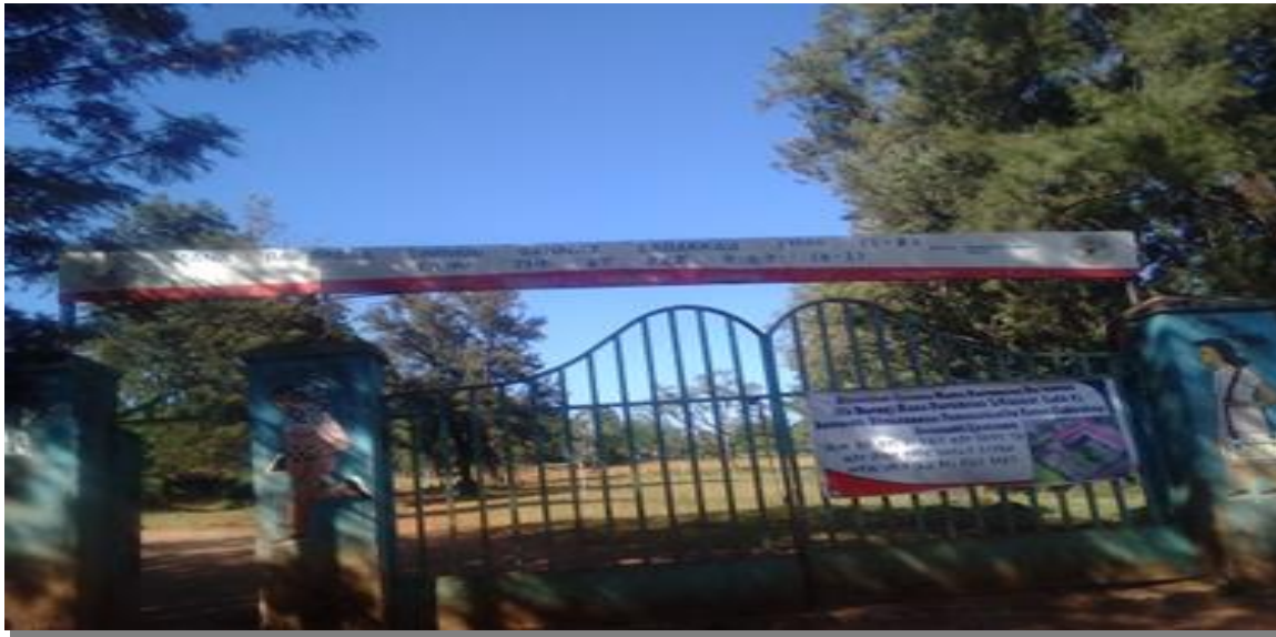
Figure 1: Limmu Genet Elementary School Built by the Swedish Aid ESBU in 1970
