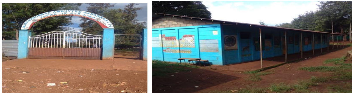
Figure 2: Ambuye Elementary School Built by the Swedish Aid ESBU in 1971
