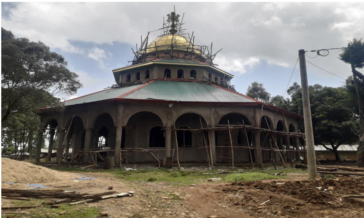
Figure 6. The construction of Yadota St.Mary church replaces of old
