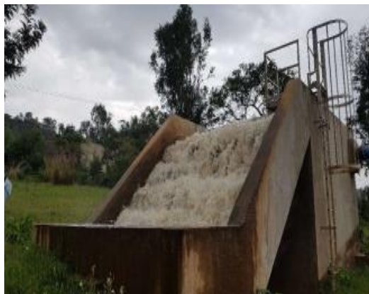
Figure 3. 4 Raw water (Photo taken by the researcher)
