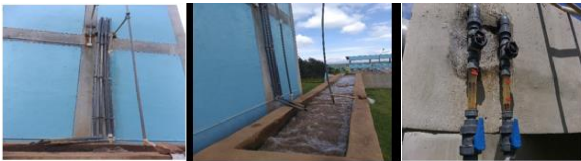
Figure 3. 3 Chemicals rapid mixing in new and old WTP (Photo taken by the researcher)
