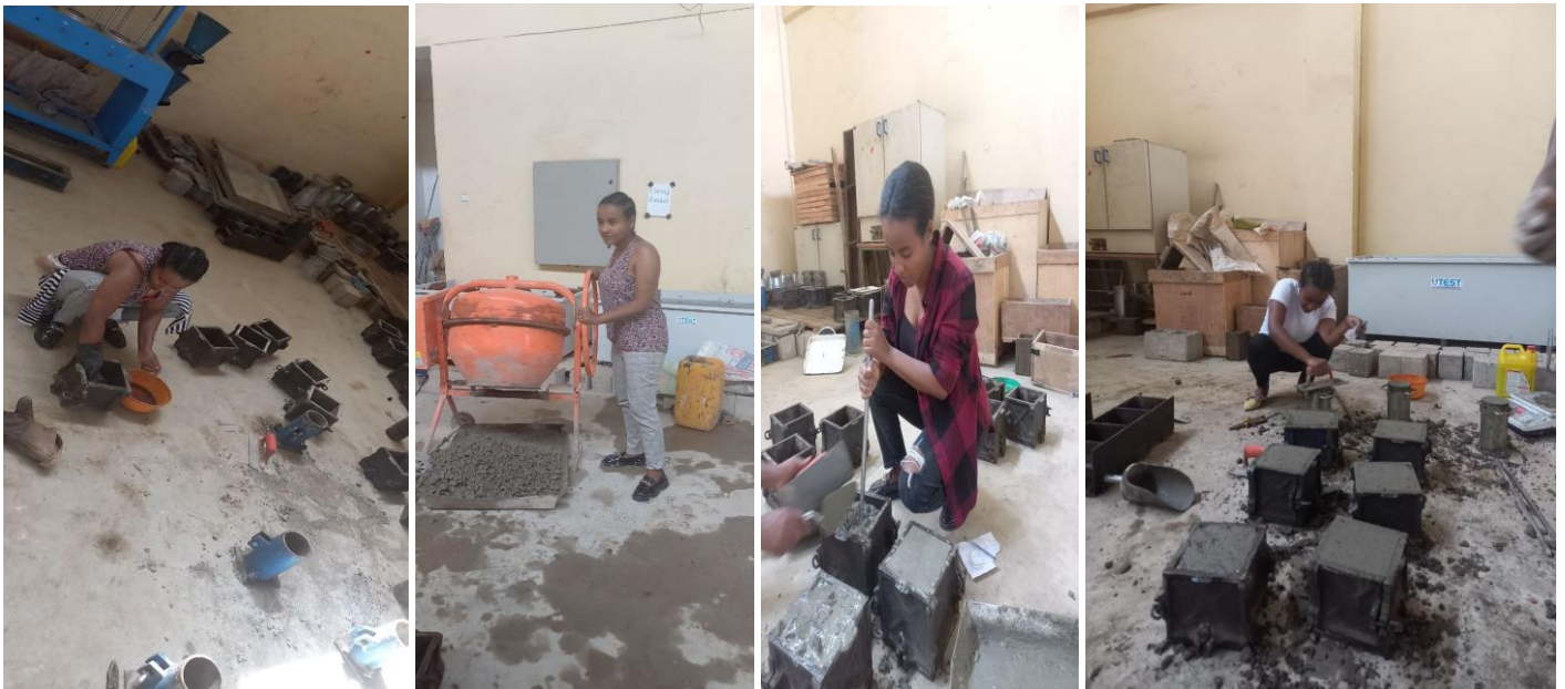
Photo-6 Prepared molds, Mix and casting
