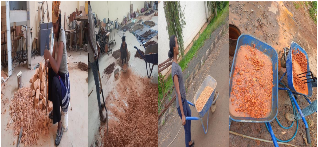
Photo-2 Crushing, sieving, transporting and washing waste brick
