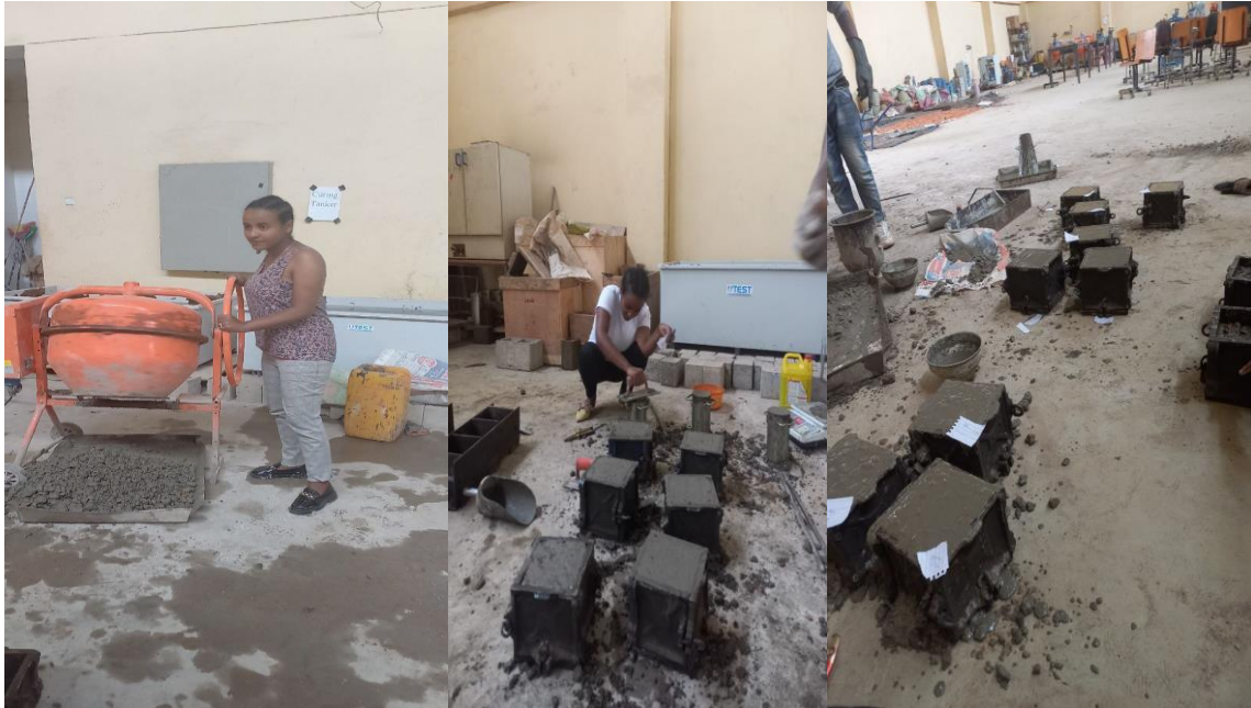
Figure 3-6 Casted concrete molds
