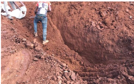
Test pit logging
