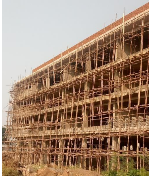
Figure 2-1 double layered eucalyptus scaffold- Teppi construction site-author
