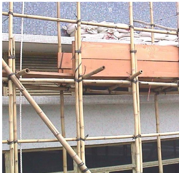
Figure 2-2 Double layered bamboo scaffold (Chan & Chung, 2002)
