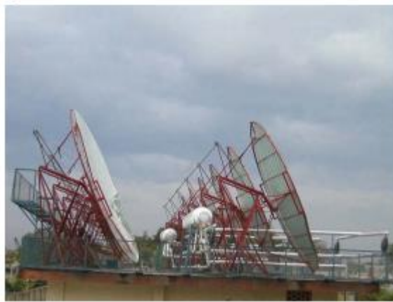
Fig. 11. Steam for dry cleaning and laundry for Gajaraj Cleaners, in Ahmadnagar, Maharashtra, India.
